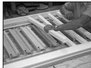
Insert 18 balusters (8' section) less for shorter section.
