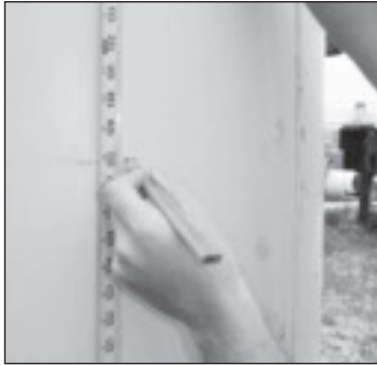
1. Measure and mark finished porch height.
