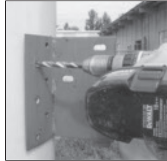
3. Using bottom mark, locate top outside hole and drill 1/2" hole.
