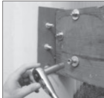
8. Apply required framing using all thread rod, washers and nuts. (See note 4) Repeat steps 1-8 for remaining two brackets. (See note 1) in lieu of 4)
