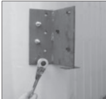
7. Drill remaining holes and tap in remaining anchors and secure. (Refer to note 4 and tips.)
