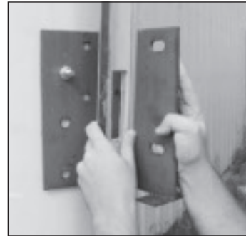
6. Level bracket and drill remaining 5 holes.
