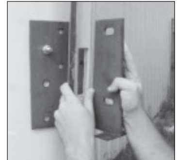
6. Level bracket and drill remaining 5 holes.
