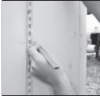
1. Measure and mark finished porch height.
