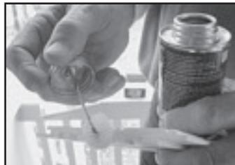
6. Use clear PVC cement where plank ends must be butted together.
