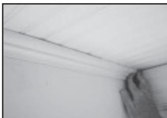
11. Trim with your choice of PermaPorch® Ceiling Molding. Install using finish nail or screws. Glue joints with PVC glue and finish with latex caulk.
