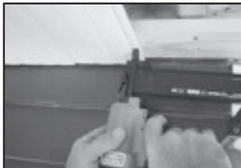
5. Optional fastening method. 16 gauge pneumatic nailers or staples are acceptable for steps two and three. Recommend PSI 75-80.
