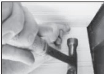
2. With the nailing fin positioned away from the wall, face nail the first piece against one side of the ceiling.
