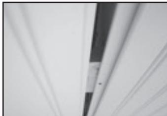
4. Insert the next piece into the slot and continue nailing through the fin on maximum 24" centers until ceiling is completely covered.
