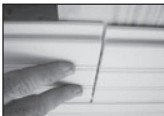
7. Make sure butt joints occur on nailers, secure each end to nailer.
