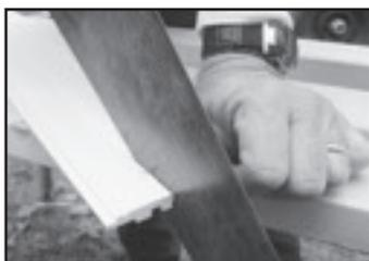
8. The last piece will probably need its width adjusted. Measure, mark and rip to the desired width.
