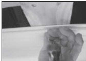
3. Nail the nailing fin on the first piece on maximum 24" centers. (See note 1)
