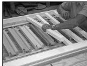
Insert 18 balusters (8' section) less for shorter section.
