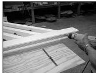
Screw top insert and bottom rail to balusters with 36 2 1/2" galvanized deck screws.
